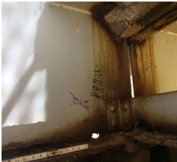
PHOTO 23 Description Span 2 at bent 3 beam 3 holes in the upper and lower webs and pitting to bottom flange up to 3/8 deep.
