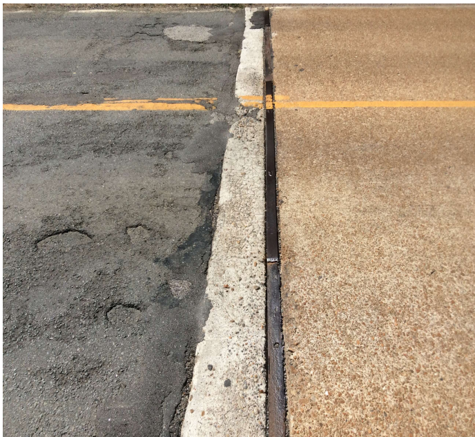
PHOTO 1 Description Bent 1, all of the sliding plate has been removed.
