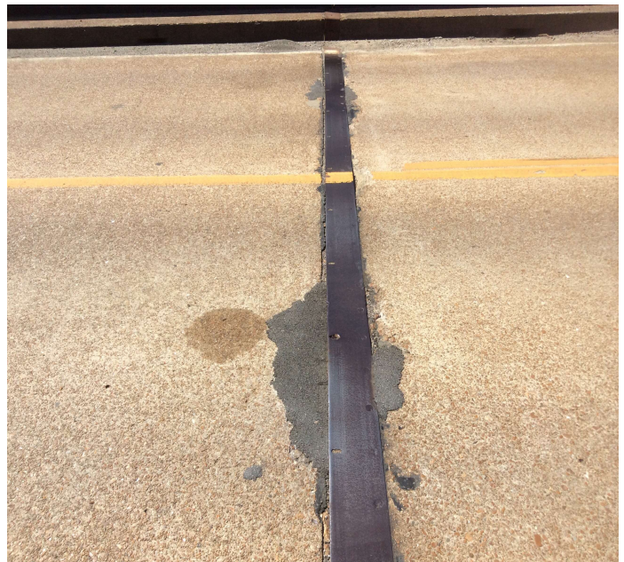
PHOTO 2 Description Bent 2, Spalls in the deck along the joint.
