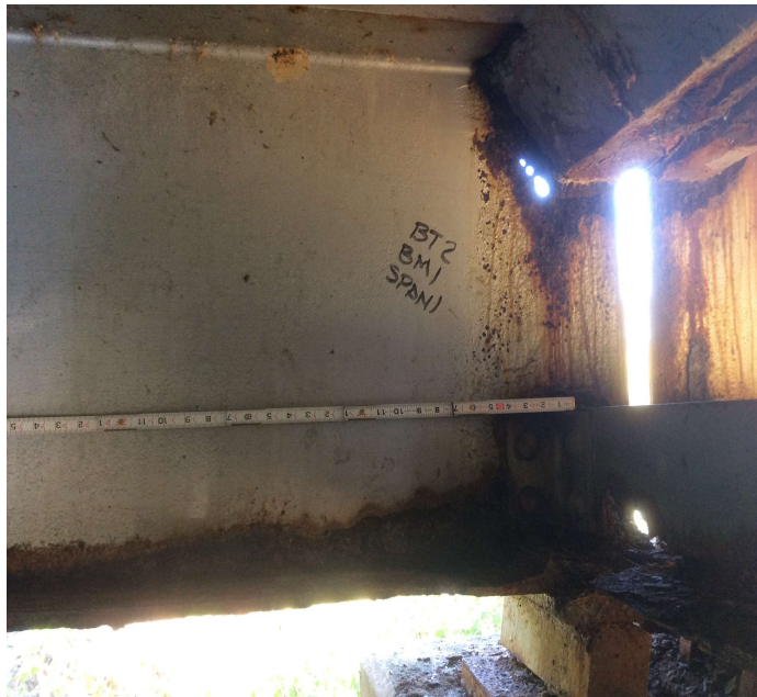
PHOTO 1 Description Span 1, beam 1, at Bent 2. Holes in the web at the deck haunch.
