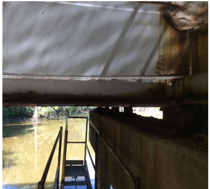
PHOTO 13 Description Span 2, beam 3 at bent 3. Hole in the upper web at haunch, Holes in the lower web back from bearing Bottom flange down to 1/2" thick x four feet both sides and Narrowed 1/2" each edge at bearing.
