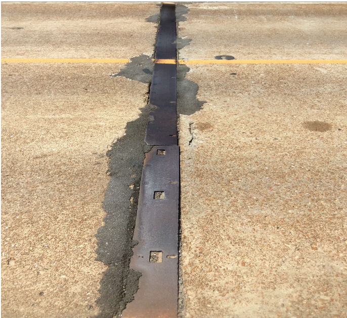
PHOTO 4 Description Assembly joint with repair at bent 4
