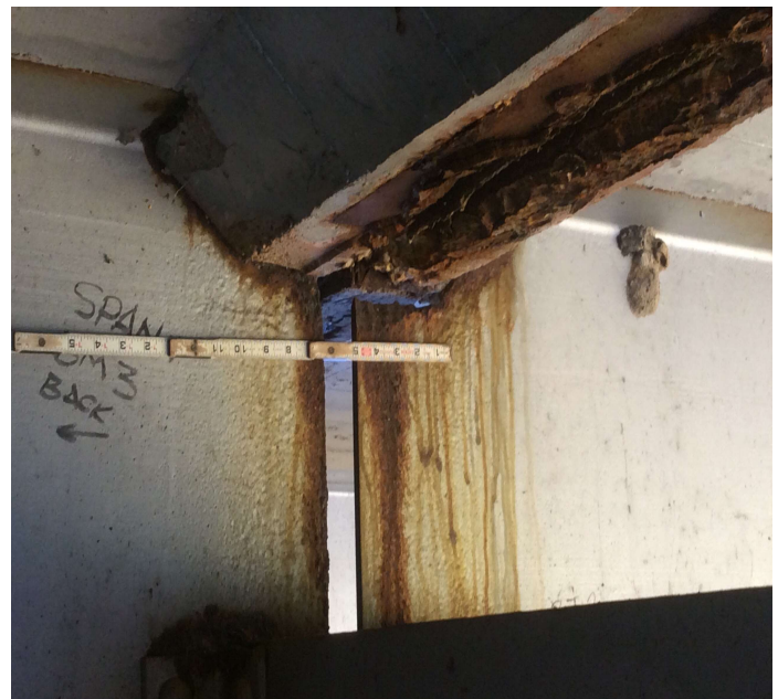
PHOTO 22 Description Bent 2 span 2 beam 3, 4 1/2" x 1" hole in upper web.
