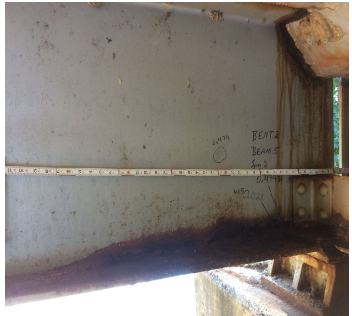
PHOTO 9 Description Span 2, beam 5 at bent 2. Pitting to 7/16" deep on the lower web, left side.
