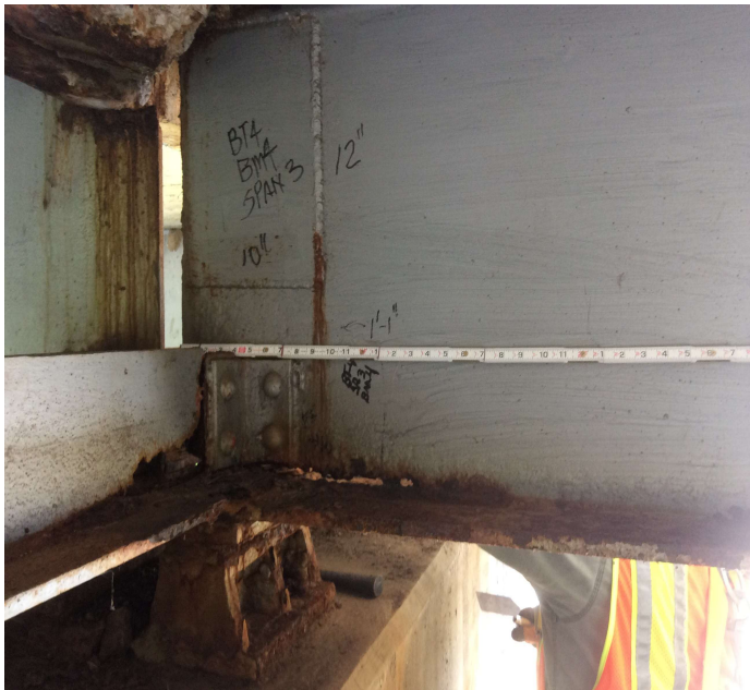
PHOTO 20 Description Span 3, beam 4 at bent 4 15" x 3/4" hole in the web at the bottom flange. Bottom flange corroded down to 3/8 thick at bearing. Repair plates at the top of the flange noted on section loss sketch.
