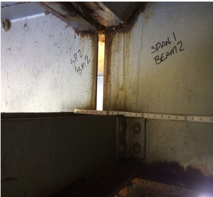
PHOTO 4 Description Spans 1 & 2 at Bent 2 Beam 2 span 1 holes in the web, span 2 beam 2, hole at the edge.
