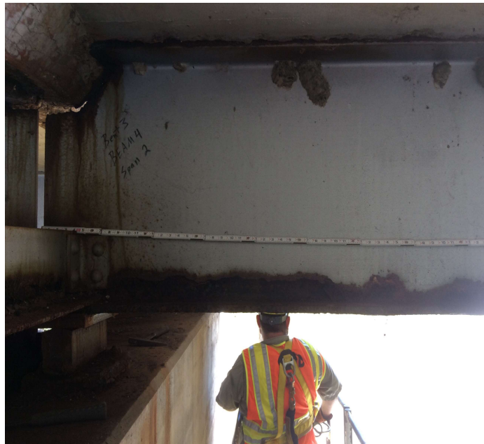
PHOTO 15 Description Span 2, beam 4, left side Hole in the web at the haunch and Pitting to the bottom flange 1/8" to 3/16" Along both sides x five feet long.
