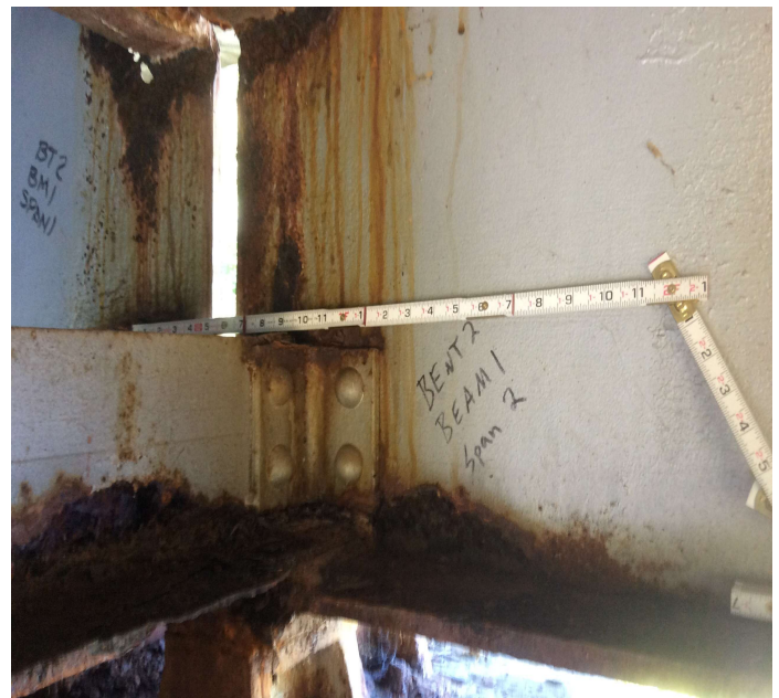
PHOTO 10 Description Span 2, beam 1 at bent 2 Pitting to the lower web 3/16" deep.
