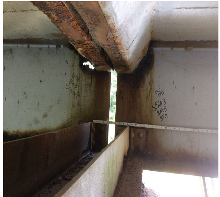
PHOTO 21 Description Spans 3 & 4 at bent 4 Beam 5 span 3 pitted to 1/4" deep at deck haunch and the bottom flange pitted to 3/16" x 1 foot back. Span 4 beam 5 hole in the web at the deck haunch.
