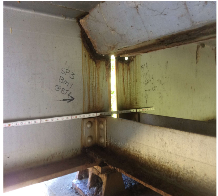
PHOTO 17 Description Spans 3 & 4 at bent 4 Beam 1 span 3 pitted at the deck haunch To 3/16" deep and lower web pitted to 1/8". Beam 1 span 4 has a hole in the web at the haunch.
