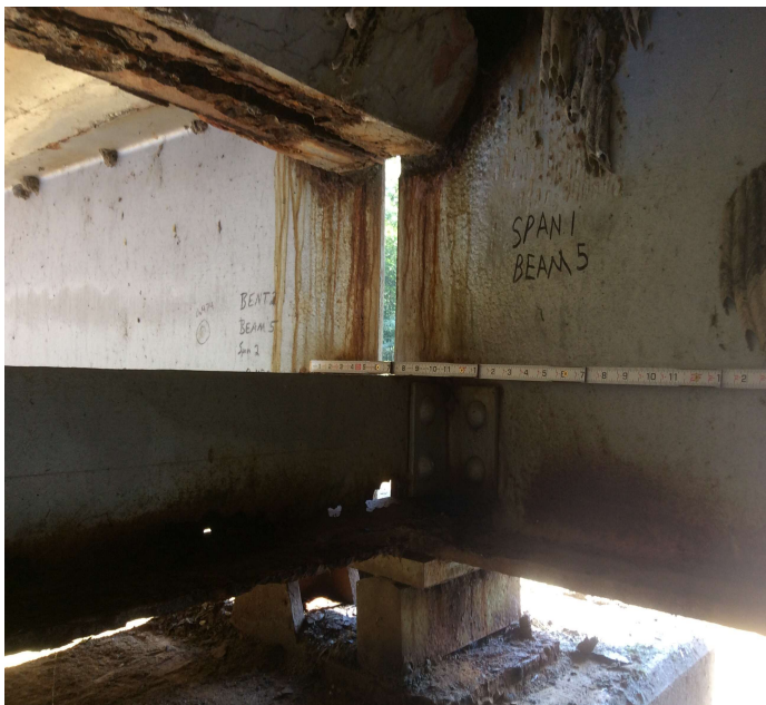
PHOTO 8 Description Span 1, beam 5, left side Pitting to 3/16" deep at the deck haunch.
