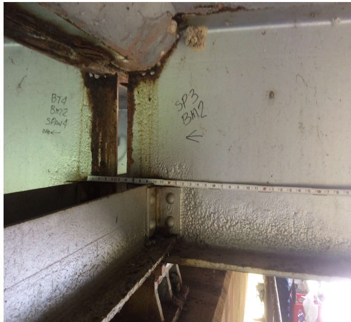
PHOTO 18 Description Spans 3 & 4, at bent 4 Beam 2 span 3 holes in the web at the haunch and Pitting to the lower web 1/8" deep x 6" tall x 2 feet. Beam 2 span 4 similar.
