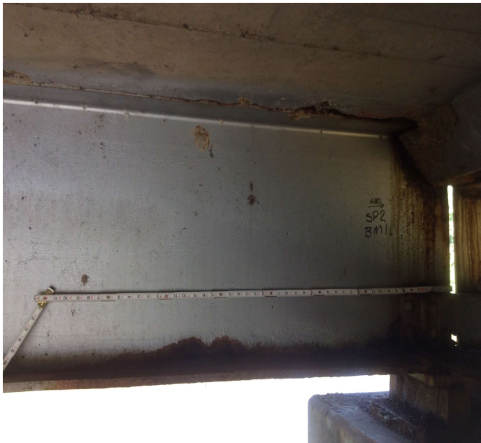
PHOTO 11 Description Span 2, beam 1 at bent 3 Pitting to 3/16" at the deck haunch and Lower web. Bottom flange pitted to 1/8" x 4 feet right side.
