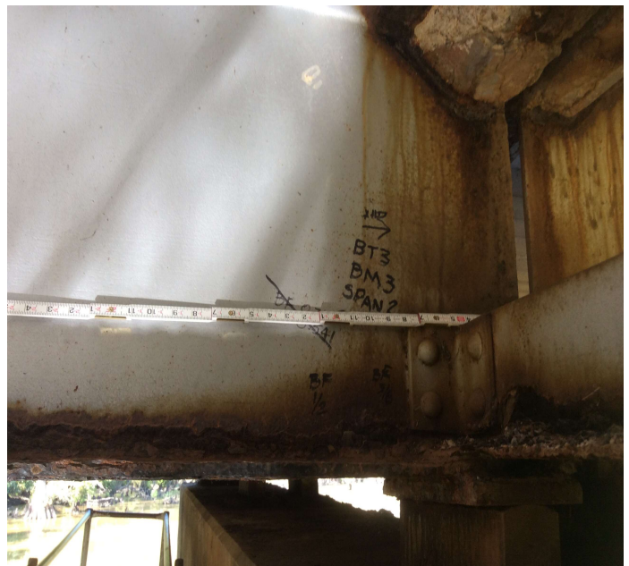
PHOTO 14 Description Span 2, beam 3 right side Closer view of holes in the web and bottom flange.
