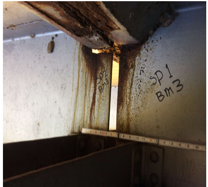
PHOTO 5 Description Spans 1 & 2, beam 3 at Bent 2 Pitting to 3/16" deep on span 1 Hole in the web on span 2.
