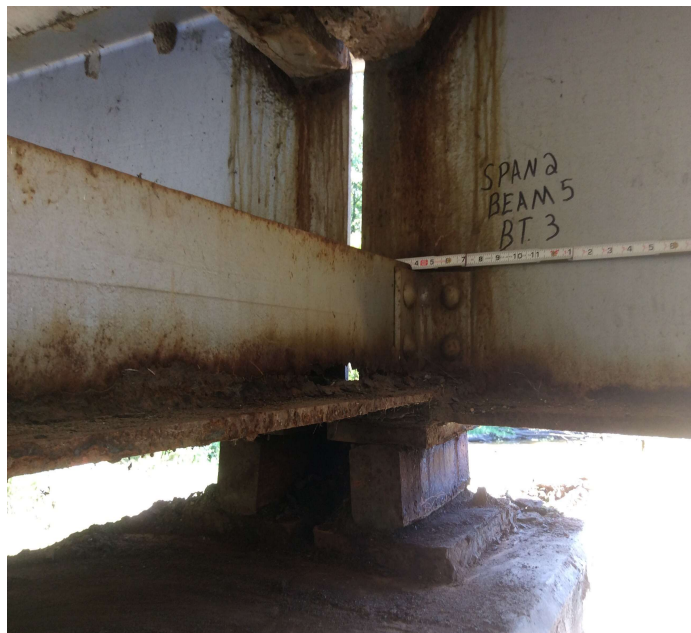
PHOTO 16 Description Span 2, beam 5 at bent 3 Pitting to 3/16" deep at haunch and The bottom flange has 1/2" remaining at bearing.
