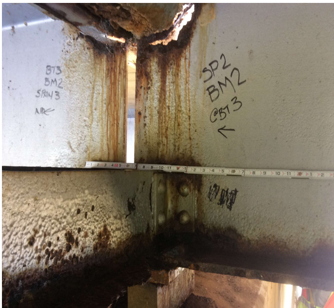
PHOTO 12 Description Span 2, beam 2 at bent 3 Hole in the web at the deck haunch and pitting to The lower web to 3/16". Bottom flange pitted to 1/8" x 1 foot back and Narrowed x 3/8" at bearing.
