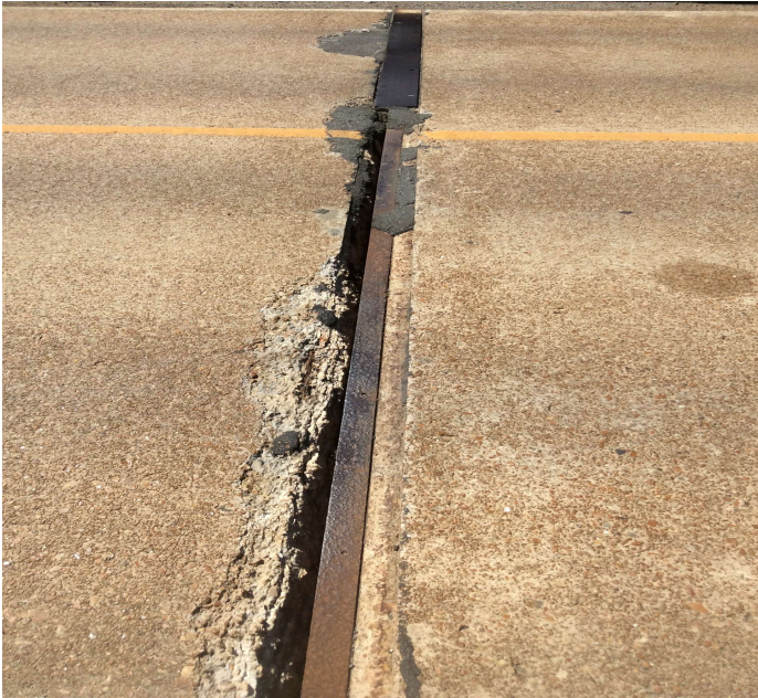
PHOTO 3 Description Bent 3, 14 feet of sliding plate is missing and the deck head steel is missing in span 2. Previous asphalt patching has failed due to joint movement. Do not use a asphalt to repair this joint.
