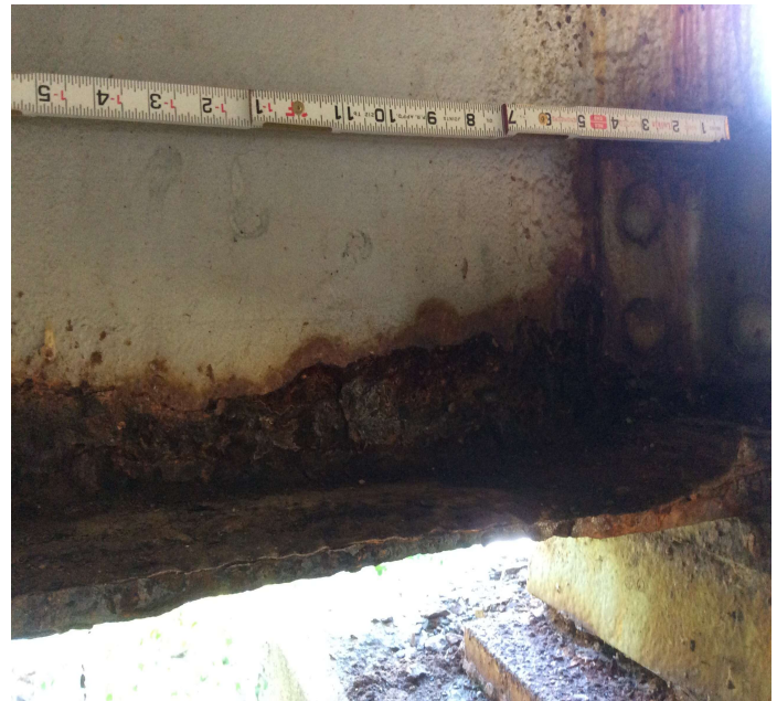
PHOTO 2 Description Span 1, beam 1, bottom flange at bent 2.
