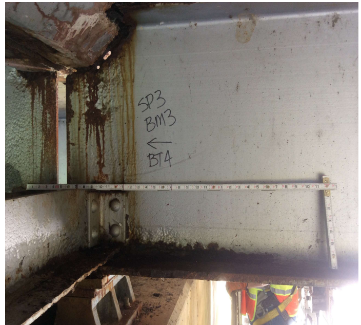
PHOTO 19 Description Span 3, beam 3 at bent 4 Holes in the web at the deck haunch and Pitting to 1/8" deep x four inches tall x two feet long to the lower web and bottom flange.
