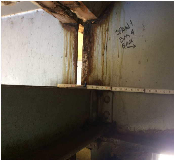
PHOTO 7 Description Span 1, beam 4 at Bent 2 Holes in the web at the haunch. Span 2, beam 4 pitted to 3/16" at haunch.
